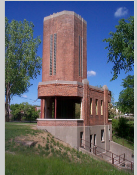
Pettibone Creek Hydroelectric Station
